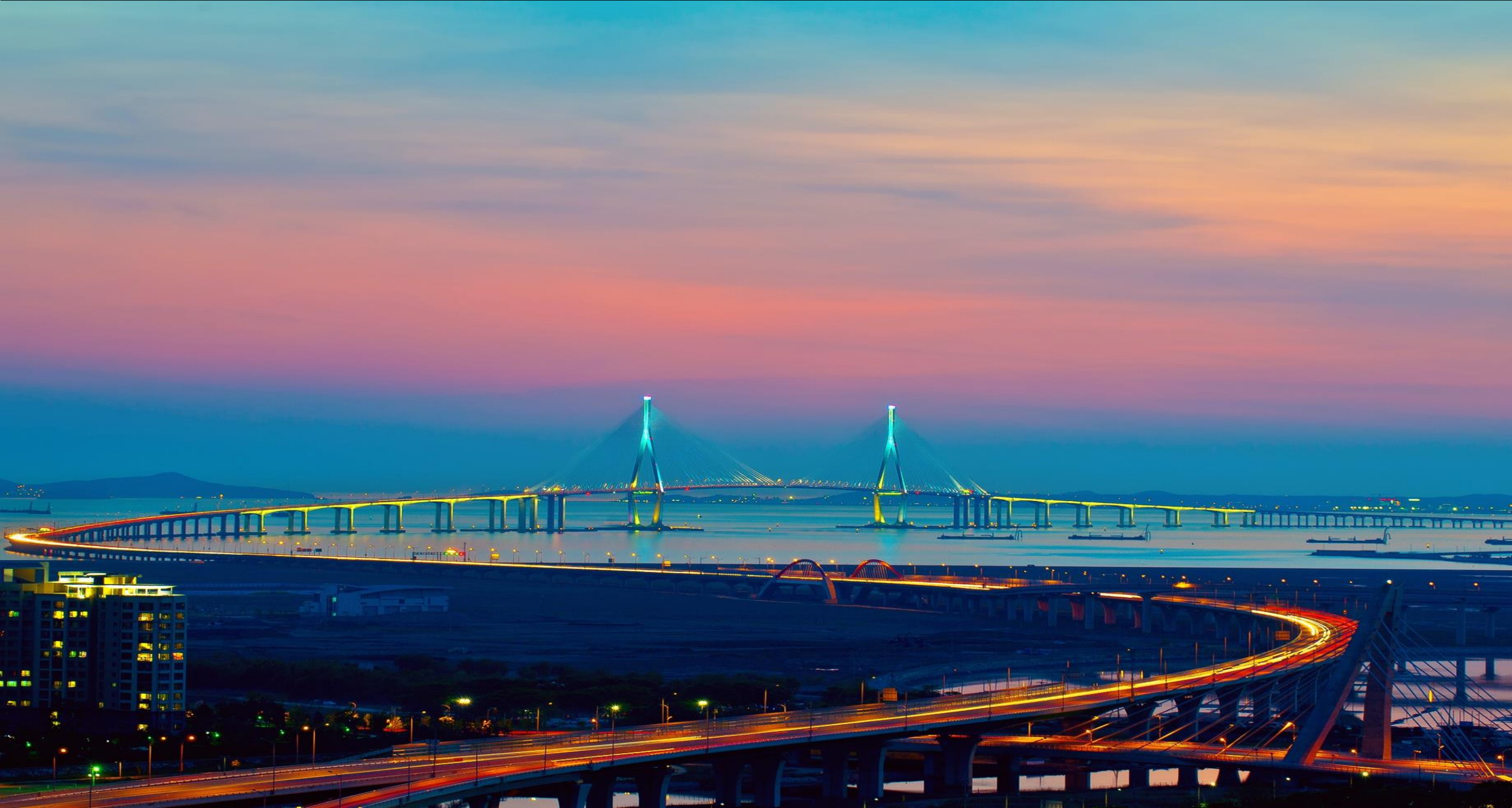
Incheon Bridge, Korea
